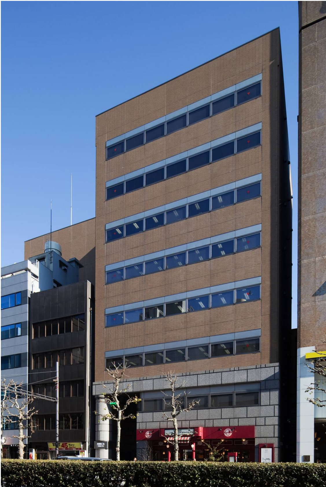
(Reference) Photo: Outside view of Kyodo Building (Kayabacho 2Chome)
