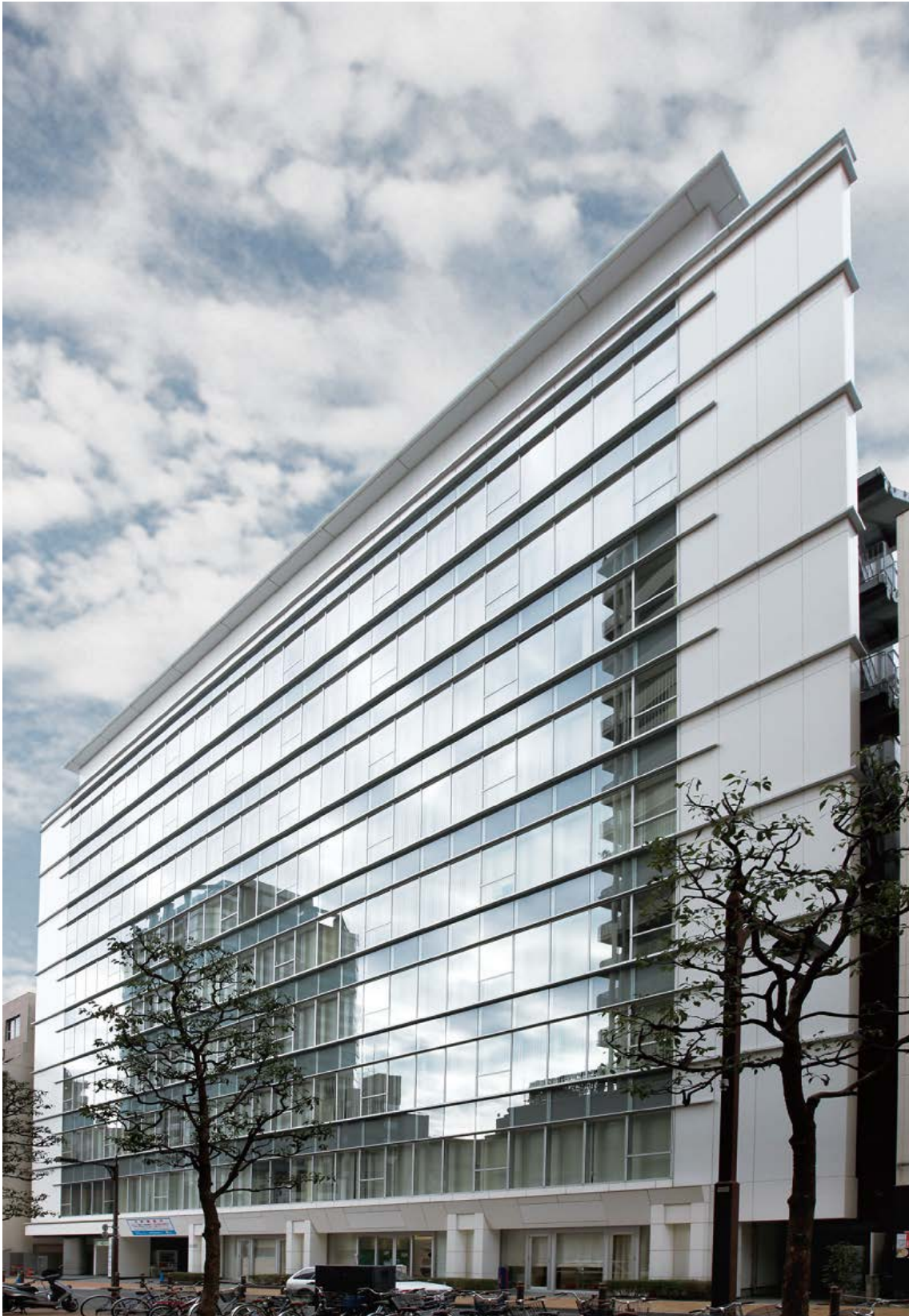
(Reference) Photo: Outside view of Ginza Ichome East Building
