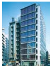
MD Kanda Building
