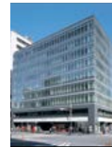
Sanno Grand Building
