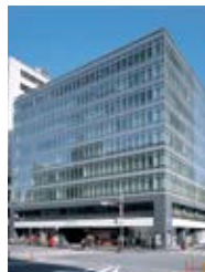
Sanno Grand Building
