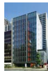
Tamachi Front Building
