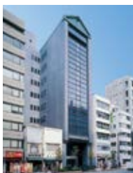
Kodemacho Shin-Nihonbashi Building
