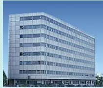
Otsuka Higashi-Ikebukuro Building
