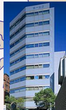
Kobe Itomachi Building
