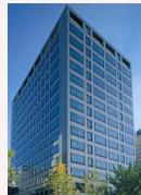
Midosuji Daiwa Building
