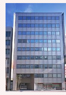
Kanazawa Minamicho Building
