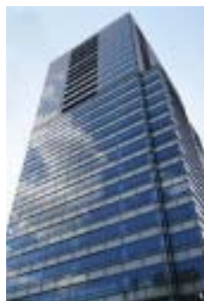
External facade (under construction)
