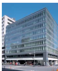
Sanno Grand Building
