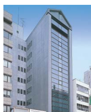
Kodenmachi Shin-Nihonbashi Building
