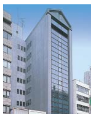
Kodenmachi Shin-Nihonbashi Building
