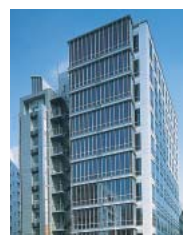
MD Kanda Building
