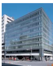
Sanno Grand Building
