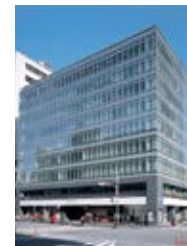
Sanno Grand Building
