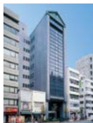
Kodonmachi Shin-Nihonbashi Building
