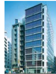
MD Kanda Building
