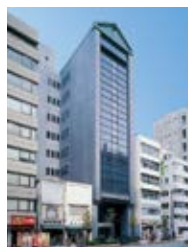
Kodonmachi Shin-Nihonbashi Building
