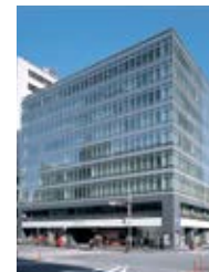
Sanno Grand Building
