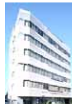
JAL Sales Building
