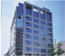
Kandabashi Park Building
