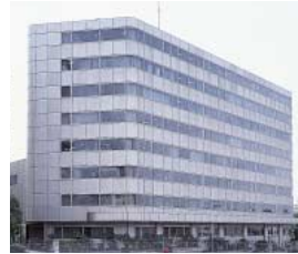
Otsuka Higashi-Ikebukuro Building
