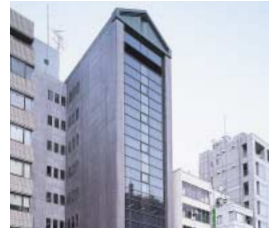
Kodenmachi Shin-Nihonbashi Building
