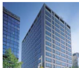
Midosuji Daiwa Building
