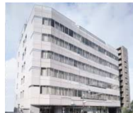
JAL Travel Building
