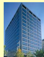
Midosuji Daiwa Building
