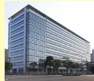
Harumi Center Building
