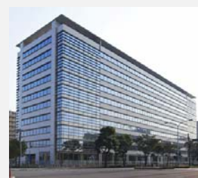
Harumi Center Building
