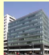
Sanno Grand Building
