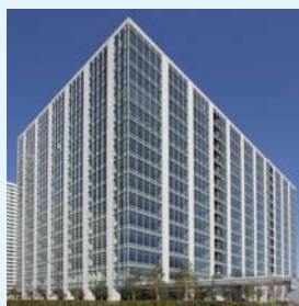
MM Park Building
