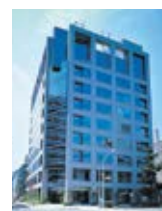
Kandabashi Park Building
