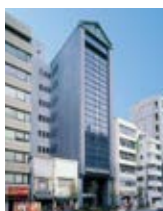
Kodenmachi Shin-Nihonbashi Building
