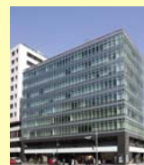
Sanno Grand Building
