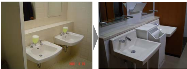
<Bathroom (Lavatory) : Before renovation> <After renovation>
