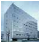
2. Niigata Ishizuecho Nishi-Bandaibashi
