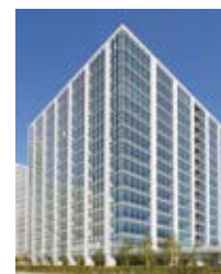
MM Park Building (Yokohama, Kanagawa Prefecture)
