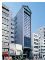
Kodonmachi Shin-Nihonbashi Building
