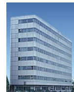
Otsuka Higashi-Ikebukuro Building
