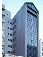
Kodenmachi Shin-Nihonbashi Building
