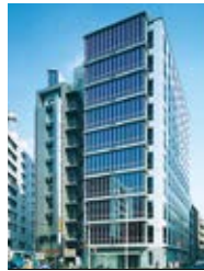
MD Kanda Building
