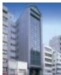
Kodenmachi Shin-Nihonbashi Building
