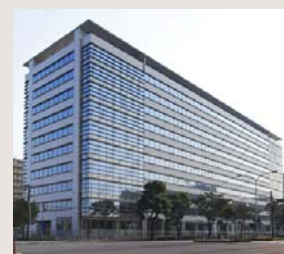
Harumi Center Building
