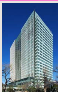
Shiodome Building (The share acquired in December 2008)
