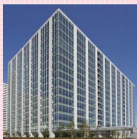
MM Park Building
