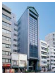
Kodonmachi Shin-Nihonbashi Building
