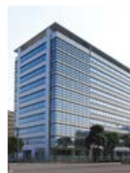
Harumi Center Building (Chuo-ku, Tokyo)
