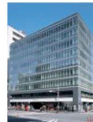
Sanno Grand Building
