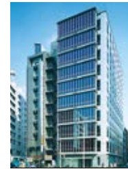
MD Kanda Building
