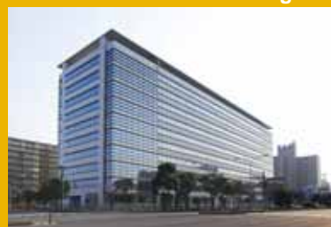
Outside view of Harumi Center Building
