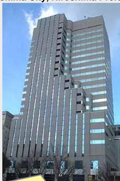
NHK Hiroshima Broadcasting Center Building (Hiroshima City, Hiroshima Prefecture)
