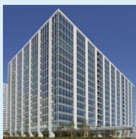
MM Park Building
