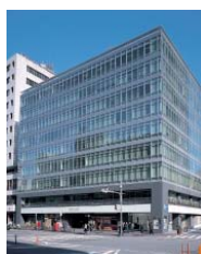
Sanno Grand Building
