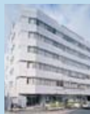
JAL Sales Building
