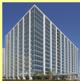
MM Park Building
