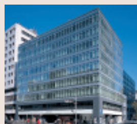
Sanno Grand Building
