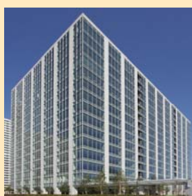
MM Park Building
