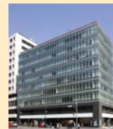
Sanno Grand Building
