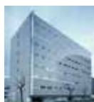
2. Niigata Ishizuecho Nishi-Bandaibashi
