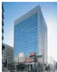
Nagoya Hirokoji Building
