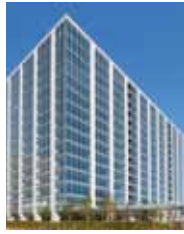
MM Park Building
