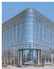
Kanazawa Park Building
