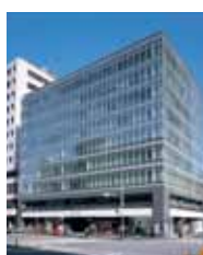
Sanno Grand Building
