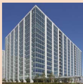
MM Park Building
