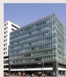
Sanno Grand Building
