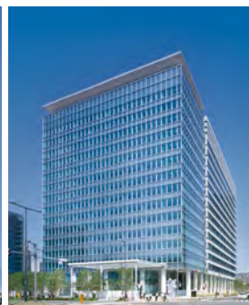
▲ Toyosu Front Transfer date: March 29, 2022 Acquisition Price: JPY 25,500 million
