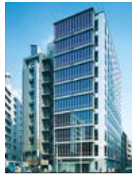
MD Kanda Building
