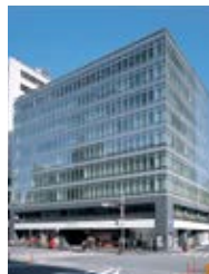
Sanno Grand Building
