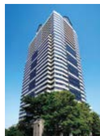
Akasaka Park Building (Minato-ku, Tokyo)
