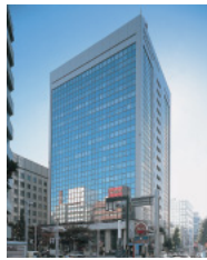
Nagoya Hirokoji Building
