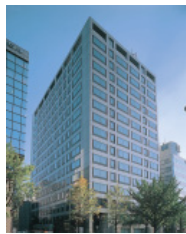
Midosuji Daiwa Building
